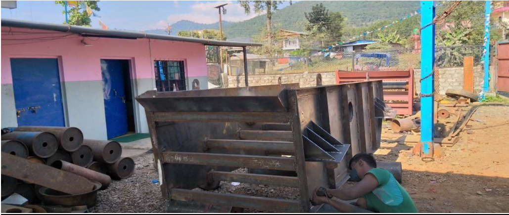
Fig: Fabrication of Crusher plant is in Progress
