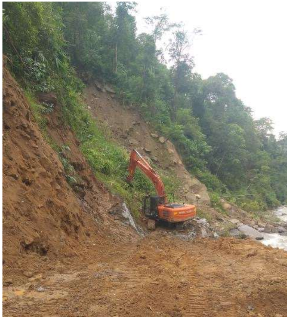
Fig: Clearing Waterway area is in Progress.
