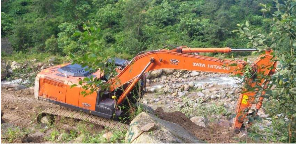
Fig: Excavation work of Waterway is in Progress.
