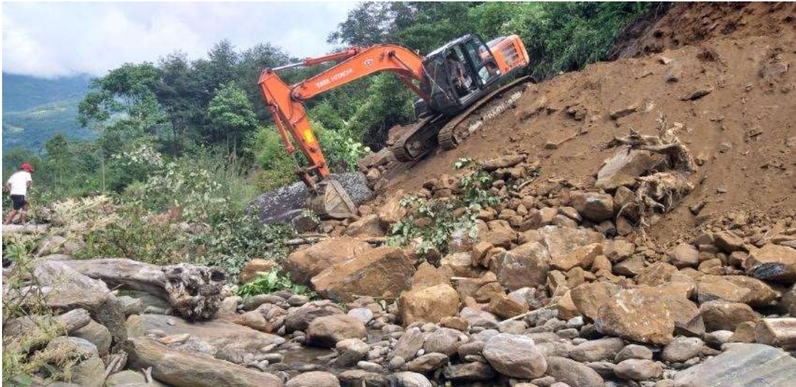
Fig: Track opening Up to Headwork
