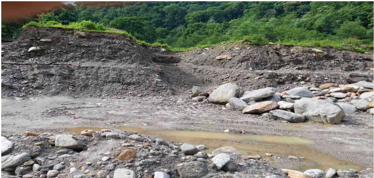
Fig: Excavation of Settling basin is in progress.
