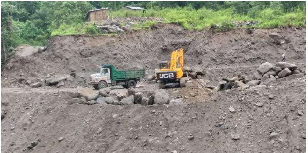
Fig: Excavation work of Powerhouse is in progress.
