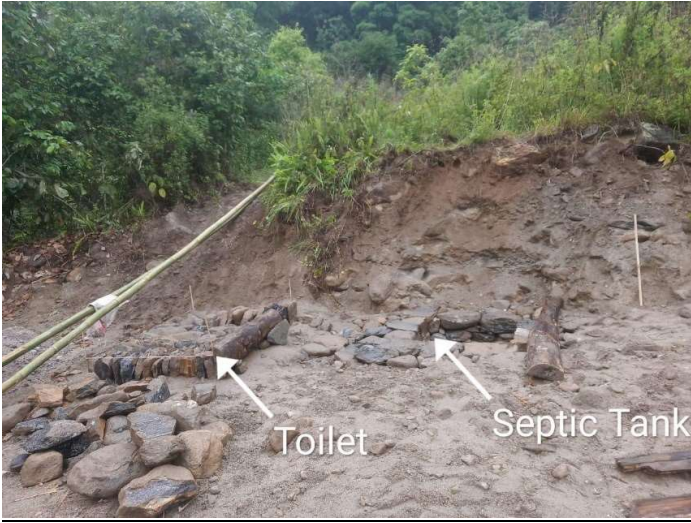
Fig: Construction of Labour Camp is in Progress
