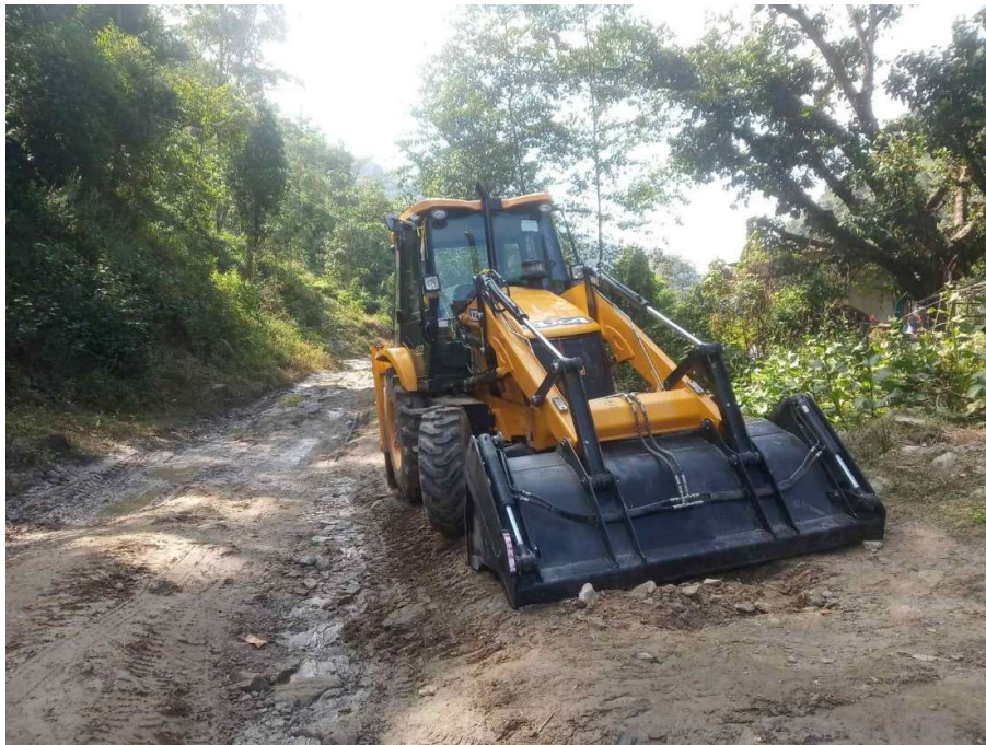
Fig: New Equipment Mobilized at Site
