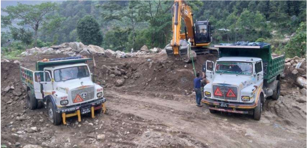
Fig: Excavation work of PH is in Progress.
